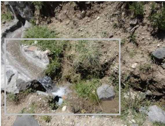
Image 19: Transition between cement and earthen sections of a partially enhanced canal. No follow-up projects are currently scheduled. Coporaque, 2013.
