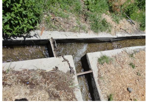
Image 96: Aerial of a cement canal and metal gates that direct the water from Santa Rosa. Coporaque, 2013.
