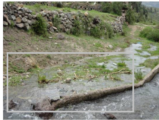
Image 18: Fissures and flooding. Coporaque, 2013.
