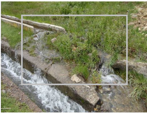
Image 17: Fissures in a cement canal. Coporaque, 2013.
