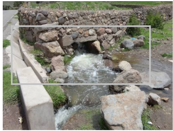
Image 20: Cement canal alongside earthen source. The initial inefficiency causes water loss and flooding. Coporaque, 2013.
